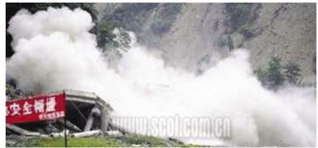
(a) Blast demolition
