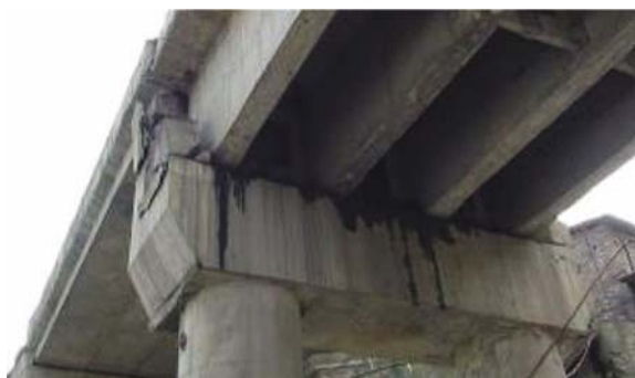
Fig. 14 Damage to shear key (left) and embankment of the overpass (right)
