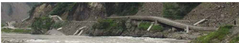
(b) After demolition
