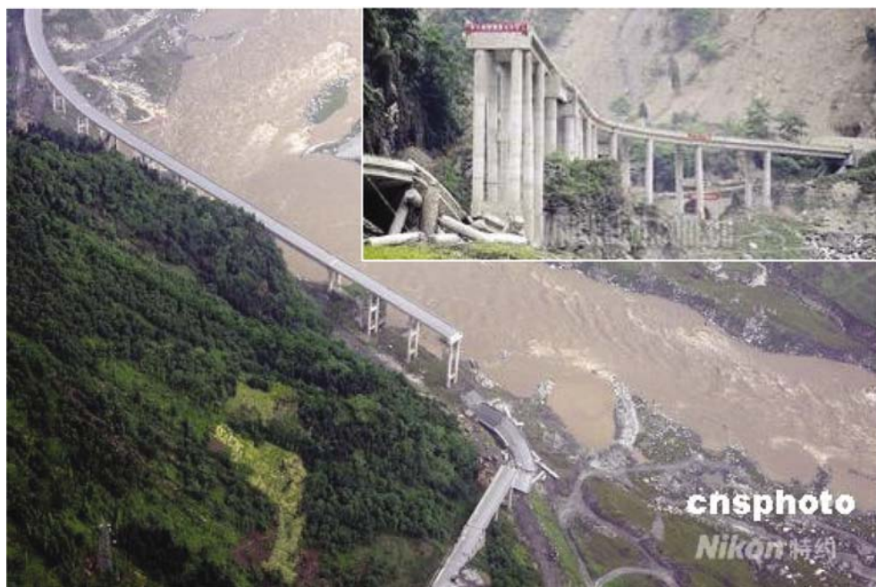
Fig. 17 Post-earthquake damage
