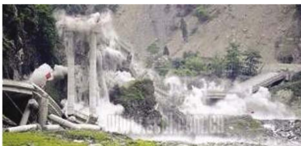
(a) Blast demolition
