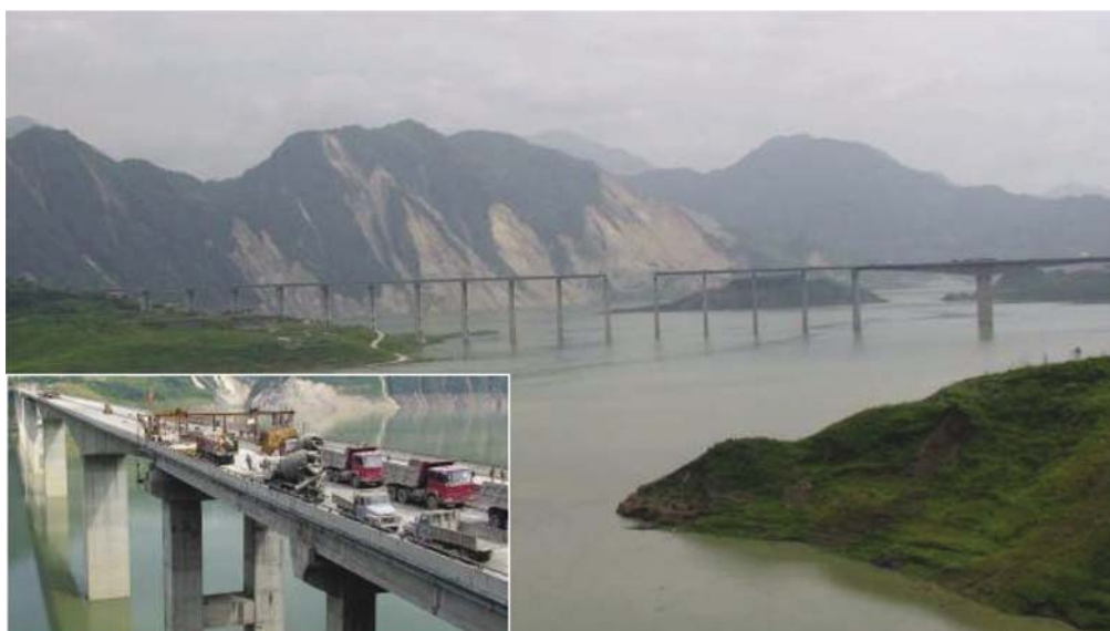
Fig. 9 Overview of the Miaoziping Bridge
