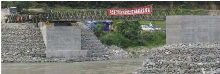
(b) Bailey bridge pushed in place
