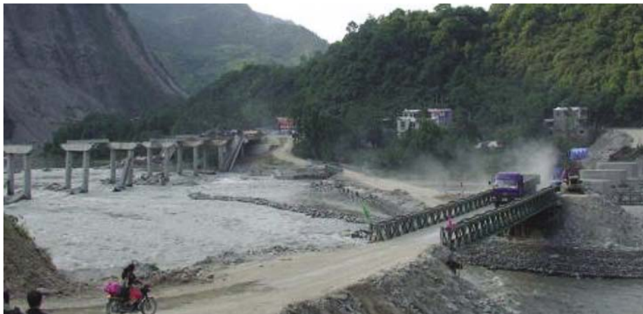
(a) Overview of a temporary bridge construction
