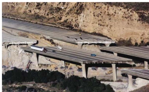
Fig. 22 I-5 Gavin Canyon undercrossing ( http://ntl.bts.gov )
