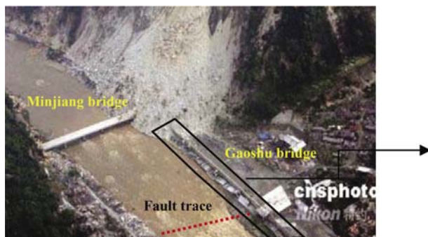
Fig. 1 Aerial view of Gaoshu and Minjiang bridges
