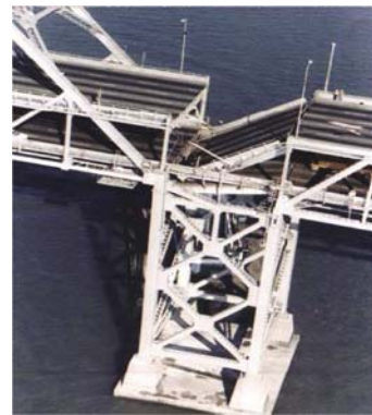
Fig. 20 San Francisco-Oakland Bay Bridge (Penzien et al. , 2003)
