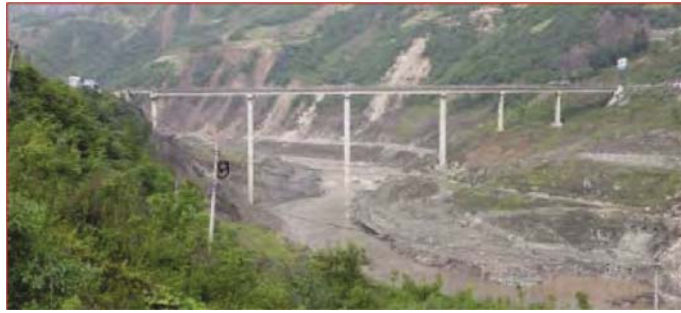
Fig. 8 Shoujiang Bridge (Li et al. , 2008)
