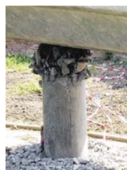
Fig. 16 Failure of column top of ramp of Huilan overpass (Yuan et al. , 2008)
