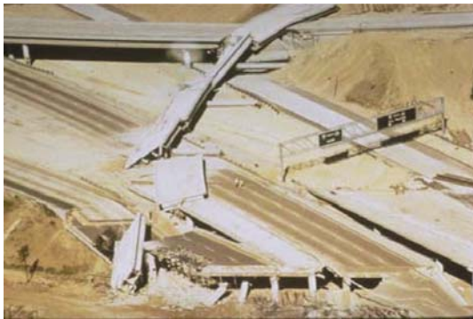
Fig. 17 Golden State Freeway (I-5) and Foothill Freeway (I-210) interchange ( http://www.smate.wvu.edu )
