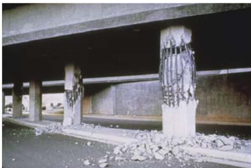
Fig. 18 Foothills Freeway overpass ( http://ntl.bts.gov )
