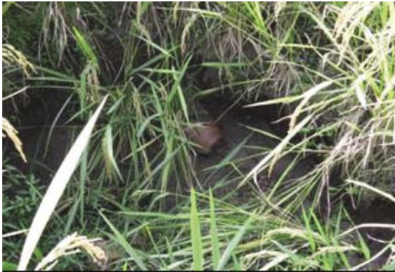
Fig. 8 Pit of 2 m in diameter caused by water spouting in Caidikan Village (Photo by ZZ Cao)
