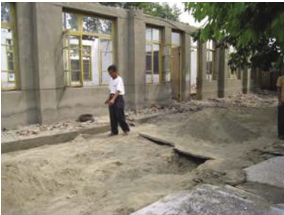
Fig. 12 Medium sand was ejected to the ground in Bilu Preliminary School and caused the destruction of the classrooms (Photo by ZZ Cao)
