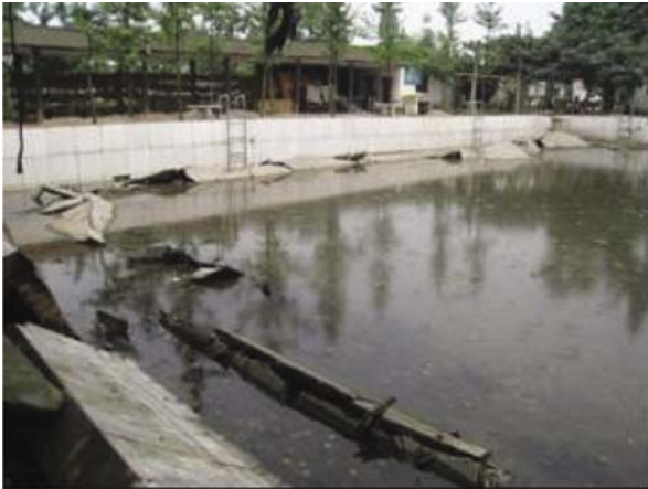
Fig. 6 Previously empty swimming pool filled with ejected sand and water of about 1m in depth after the earthquake (Photo by ZZ Cao)
