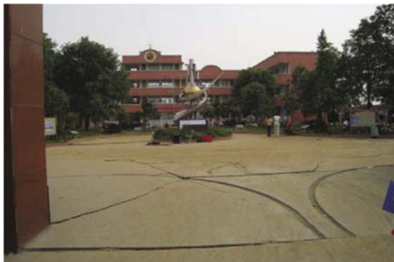
Fig. 19 Sand ejected in the school yard (left) and liquefaction-induced destruction/tilt of the main teaching building (right) of Banqiao School. (Photo by LW Chen)
