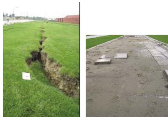
(b) Ground fissure and visible sand ejected
