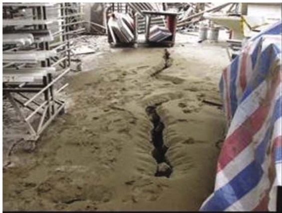
Fig. 18 Liquefaction- along with ground shaking, induced destruction to factories (Photo by ED Guo)
