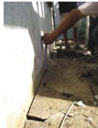
Fig. 15 Liquefaction reoccurrence following the aftershock (left) and subsidence of the house adjacent (right) (Photo by WM Wang)
