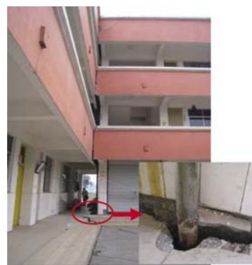
Fig. 19 Sand ejected in the school yard (left) and liquefaction-induced destruction/tilt of the main teaching building (right) of Banqiao School. (Photo by LW Chen)
