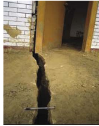
Fig. 11 Grey and yellow fine sand ejected to the ground following liquefaction behaviors (Photo by JS Bo and ZZ Cao)
