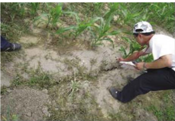
(a) Ground fissure and sand ejected
