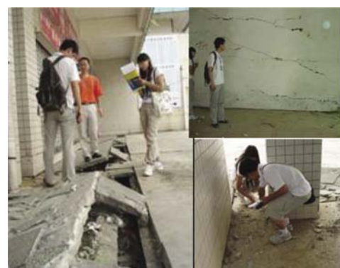
Fig. 20 Liquefaction-induced destruction of Jiangyou Railway Station along with ground shaking, including ground cracks and foundation settlement (Photo by WM Wang and L Dong)
