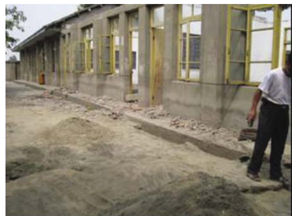
Fig. 12 Medium sand was ejected to the ground in Bilu Preliminary School and caused the destruction of the classrooms (Photo by ZZ Cao)
