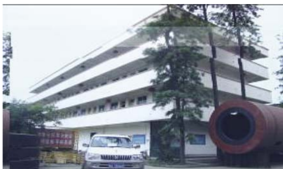
Fig. 5 Overview of RC frame office building
