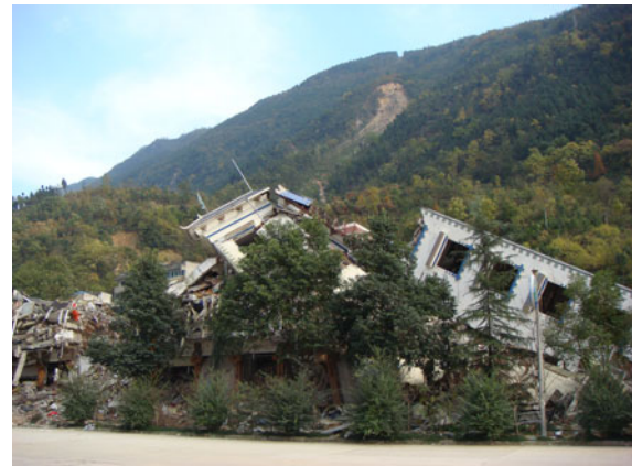
Fig. 26 Sequential collapse of commercial buildings in Beichuan County (0.1g/1.0g)
