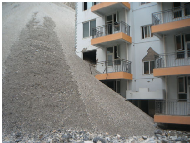
Fig. 3 Apartment building partially buried by landslide in Wenchuan County
