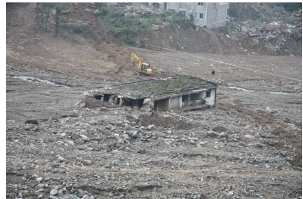
Fig. 4 Apartment building mostly buried by debris flow late Sept. in Beichuan County
