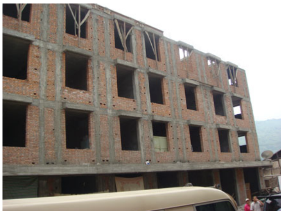
Fig. 24 Good performance of four-story confined masonry apartment building (0.1g/0.4g)
