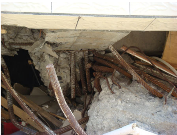
Fig. 10 Less reinforcements to column than beam (0.1g/1.0g)
