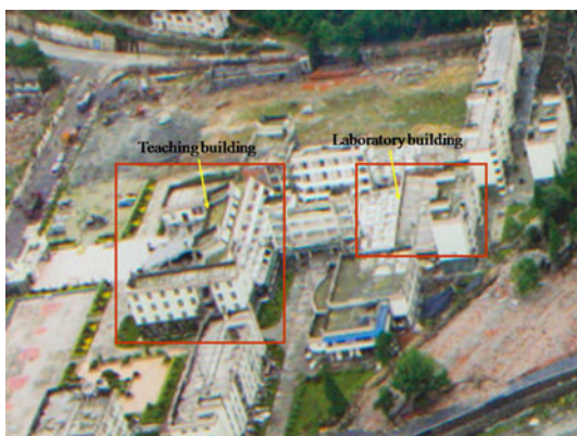
Fig. 19 Damaged Xuankou High School (0.1g/1.0g)
