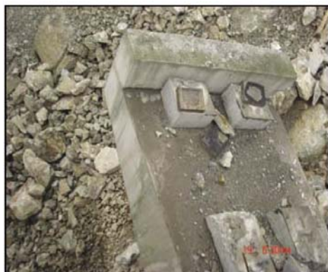
(c) Exposed bearings (at location A)
