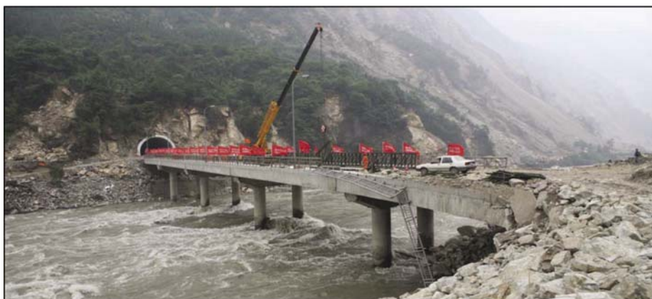
Fig. 9 Mingjiang Bridge in Yingxiu
