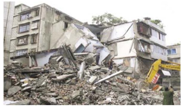
Fig. 10 Masonry residential building in Kuiyuandongjie District (Group B, collapsed)
