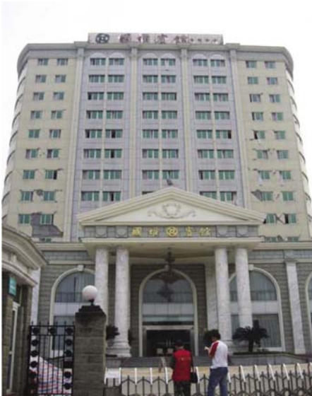
Fig. 13 RC frame structure, Guoyan Hotel (Group C, moderately damaged)
