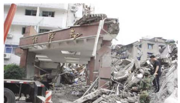
Fig. 11 Inpatient department of Hospital of Traditional Chinese Medicine (Group B, collapsed)
