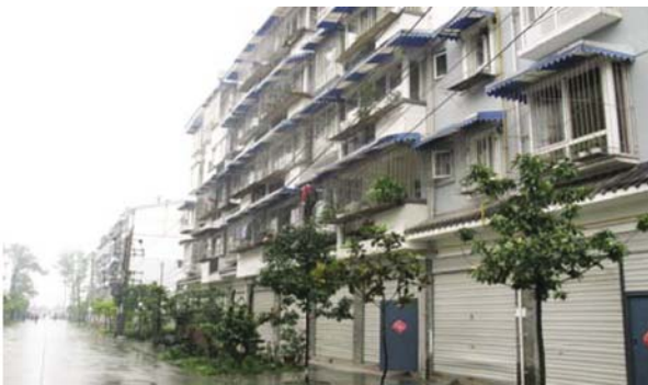
Fig. 14 Masonry residential building in Gaoqiao District (Group C, negligibly damaged)
