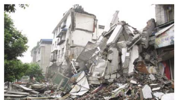
Fig. 9 Masonry structure in Hehuachi District (Group B, collapsed)
